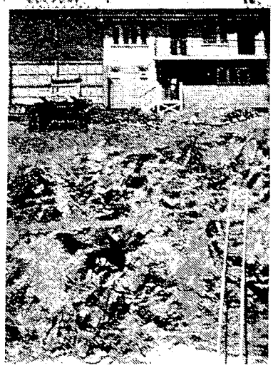
This picture shows the extensive excavations completed on the Torbreck site. At top the site office, a temporary building for use of the builders and unit owners.
